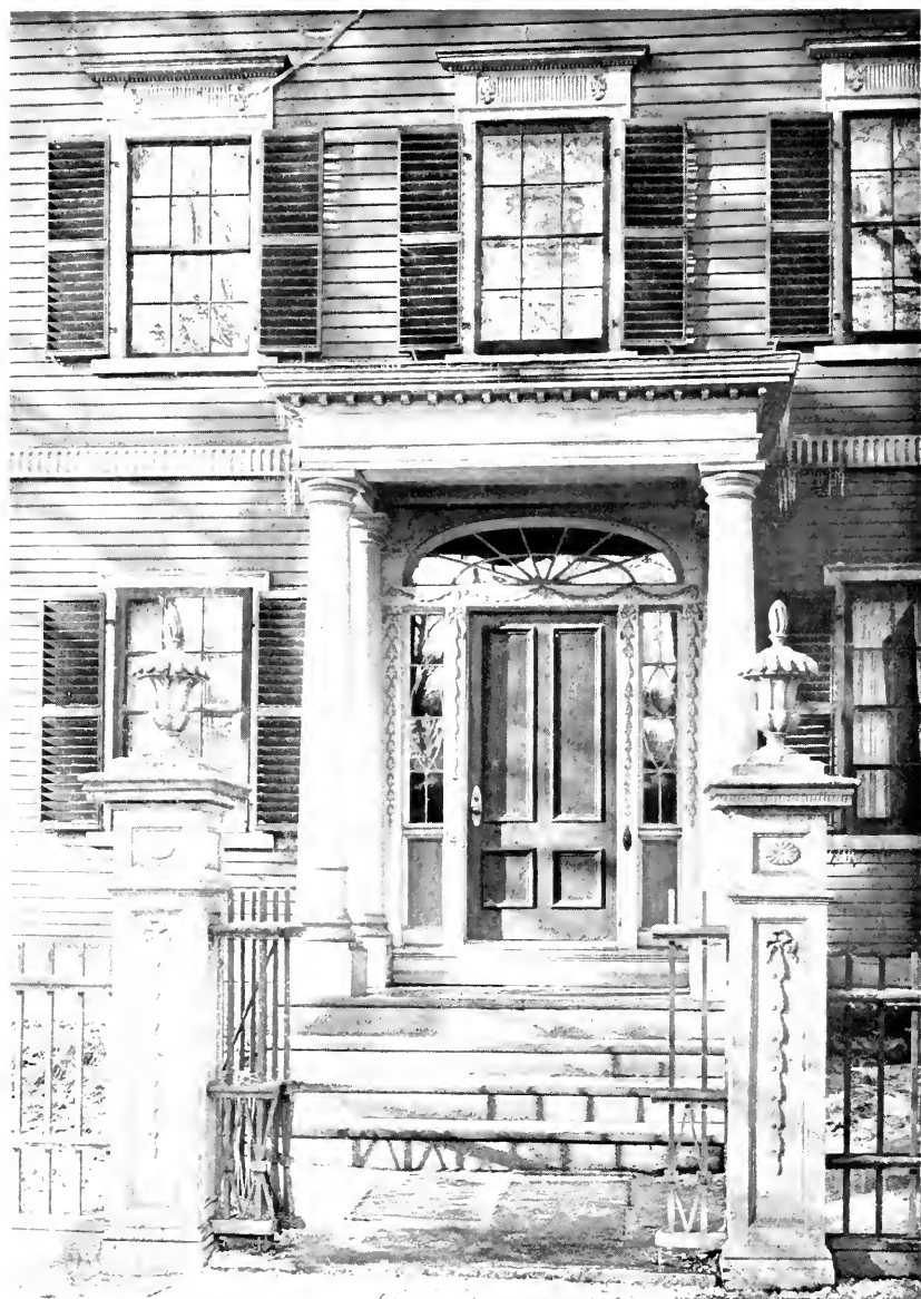
PLATE LXXVIII.—Cook-Oliver Entrance, showing Window Heads.
